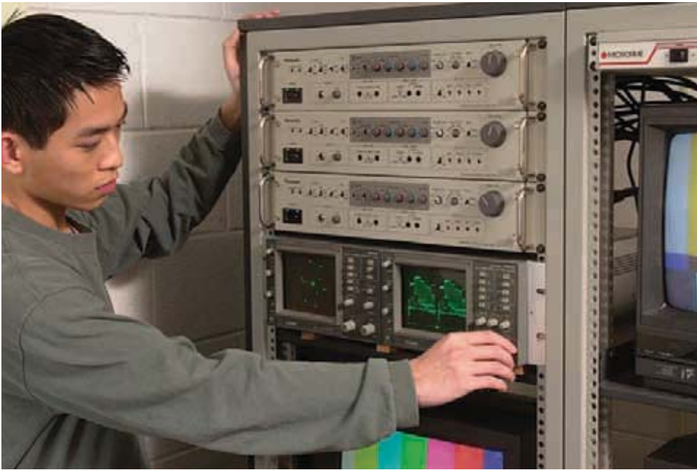
Figure 2-6. The video engineer uses specialized test equipment to examine and maintain consistent picture quality.
